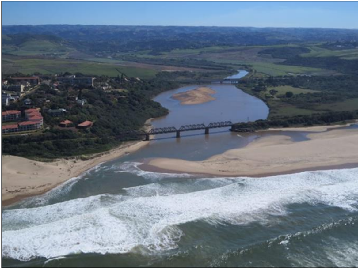
Figure 3.7. Onshore view of the iLovu Estuary, with the railway bridge across the mouth and the N2 road bridge towards the back (Coast KZN).
