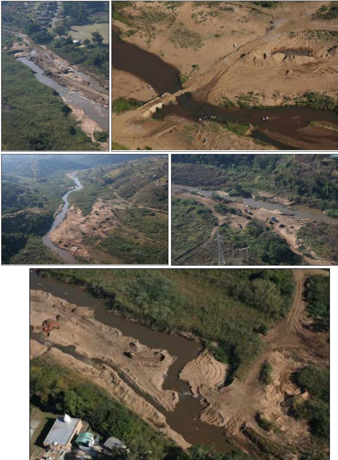
Figure 5.7. Sand mining operation on the iLovu Estuary, clearly illustrating infilling, river diversion and destruction of riverine habitat (from MER, 2007).
