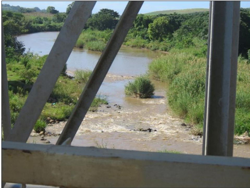
Figure 5.5. Rock Causeway just east of the 4th road bridge across the iLovu Estuary.
