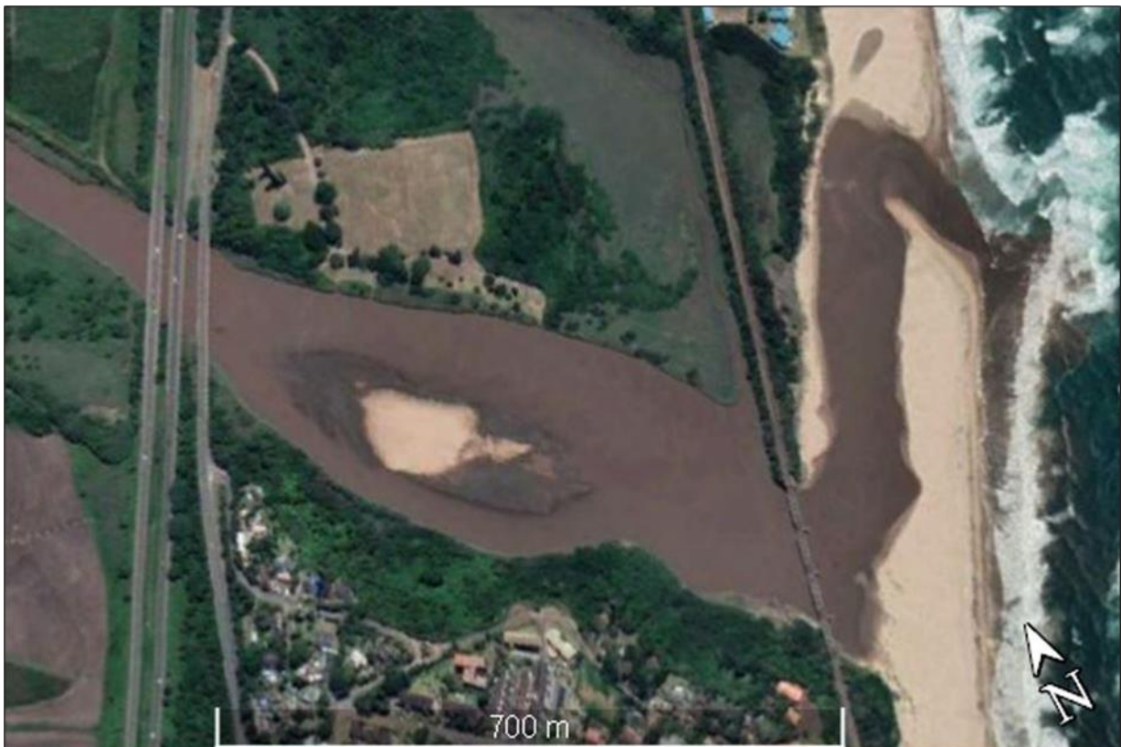
Figure 5.4. Google Earth Image (January 2021) showing the three bridges (Dual N2 & R102) and the railway line crossing the iLovu Estuary.
