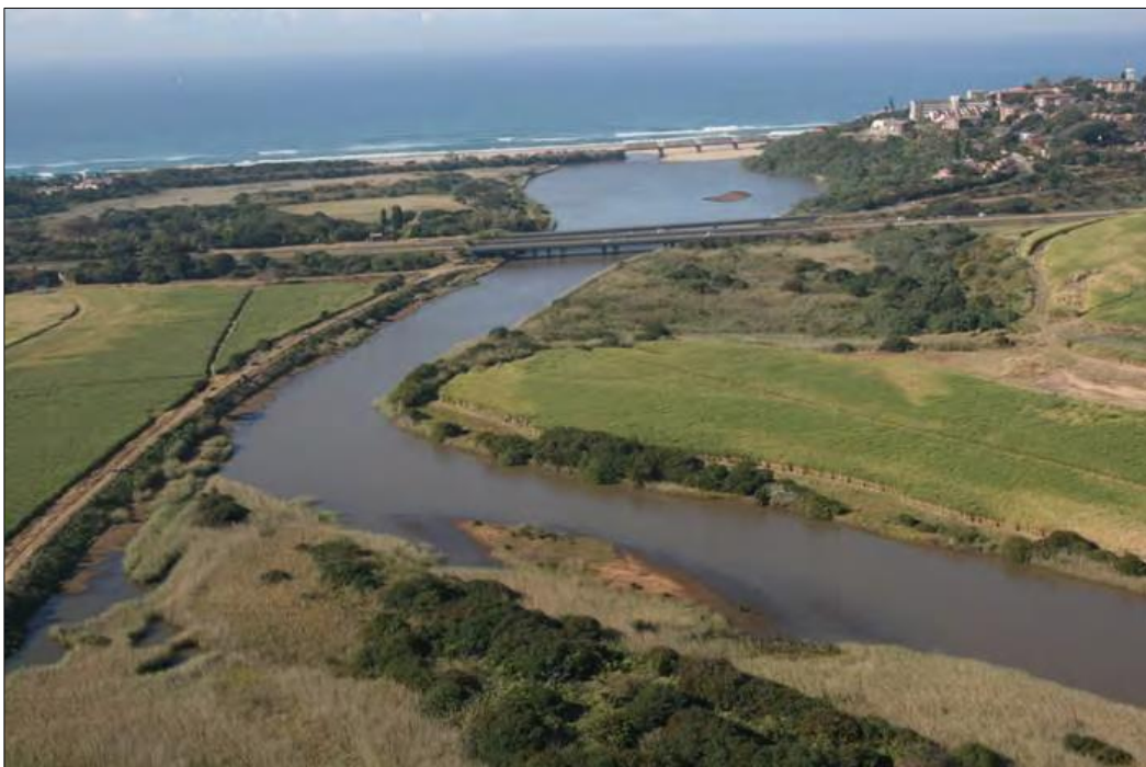
Figure 3.9. Loss of habitat /reduction of the estuarine area due to infilling and levee construction (from MER 2019a).
