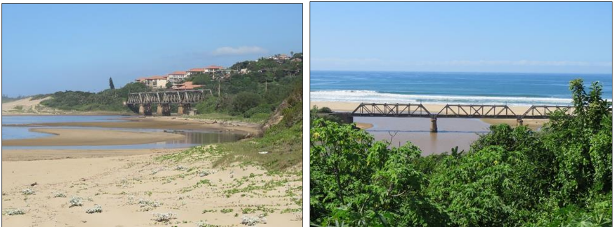
Figure 5.1. Railway bridge at the mouth of the iLovu Estuary.
