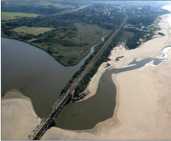
Figure 5.2. Oblique aerial showing the 500 m long causeway which has effectively removed part of the estuary (from MER 2019a).
