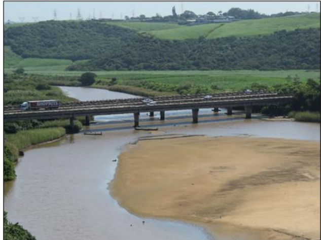
Figure 5.3. The double Bridge Dual Lane Freeway (N2) crossing the iLovu Estuary, with the old main road (R102) bridge in front of it. Note the remnant pilings of a previous bridge still in position in front of the three bridges.
