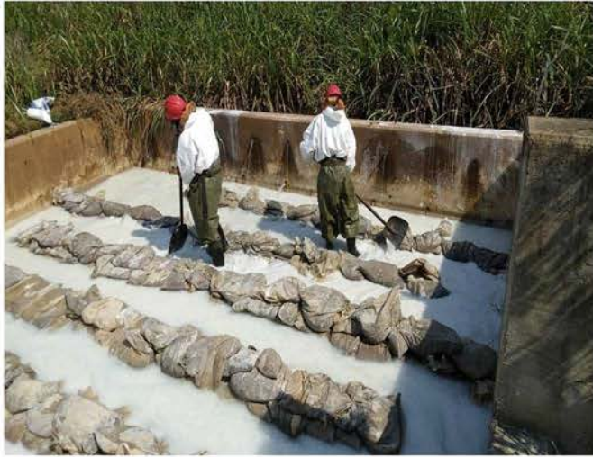
The team applying lime within the upper TD.
