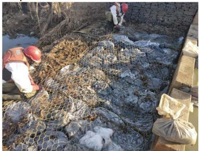
The team installing carbon bags in the gabions at Weir 1.
