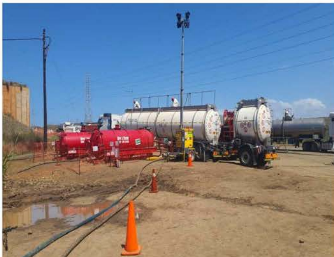
The team pumping contaminated water from the PCD into road tankers.
