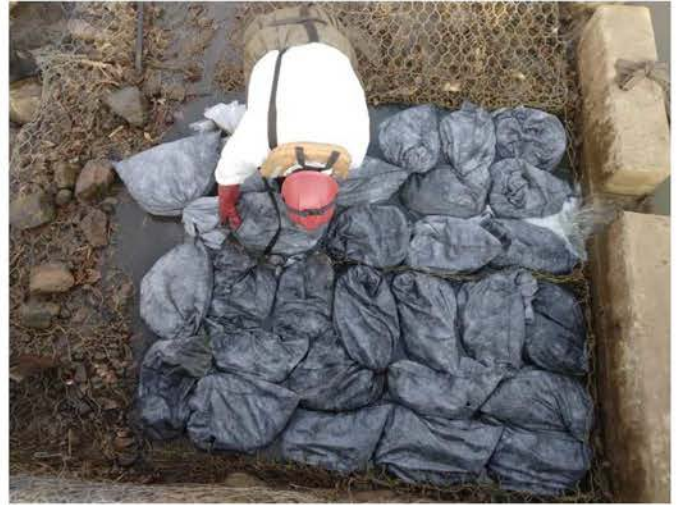
The team installing the carbon bags in the gabions at Weir 2.
