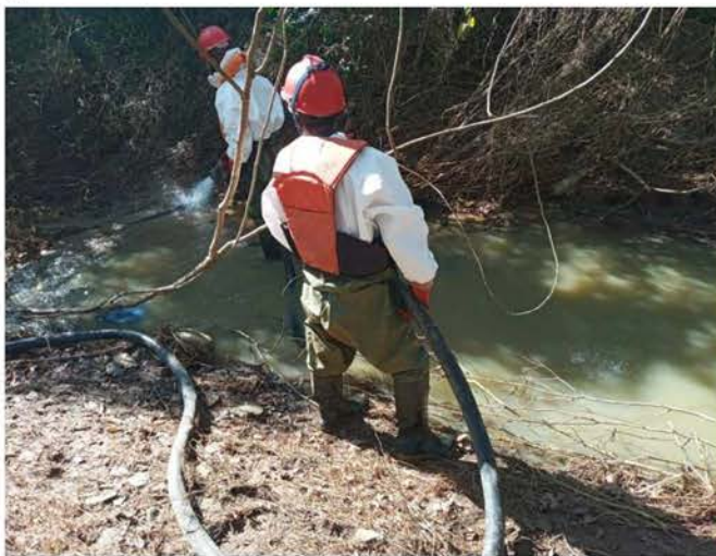
The team washing the stream with clean water.
