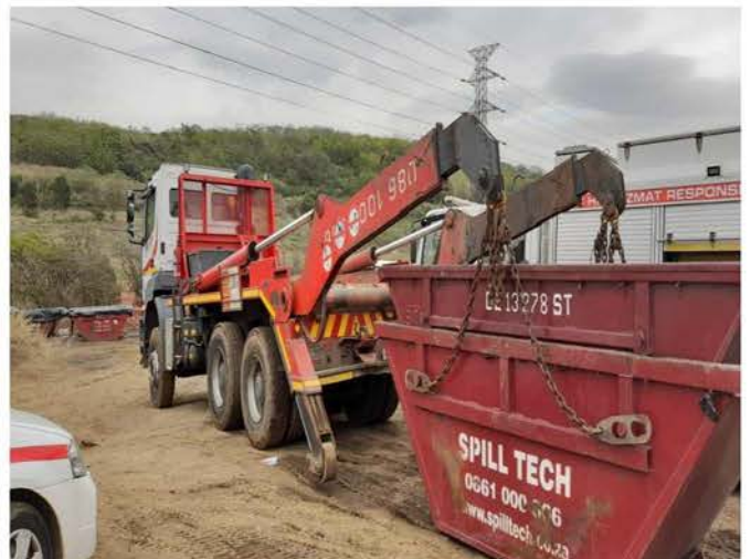
The skip truck team placing empty skip bins on site.
