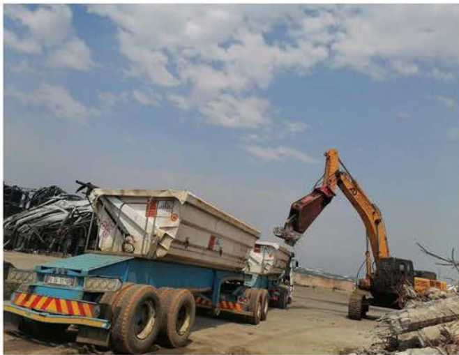
The tipper truck loading contaminated concrete in Zone D.
