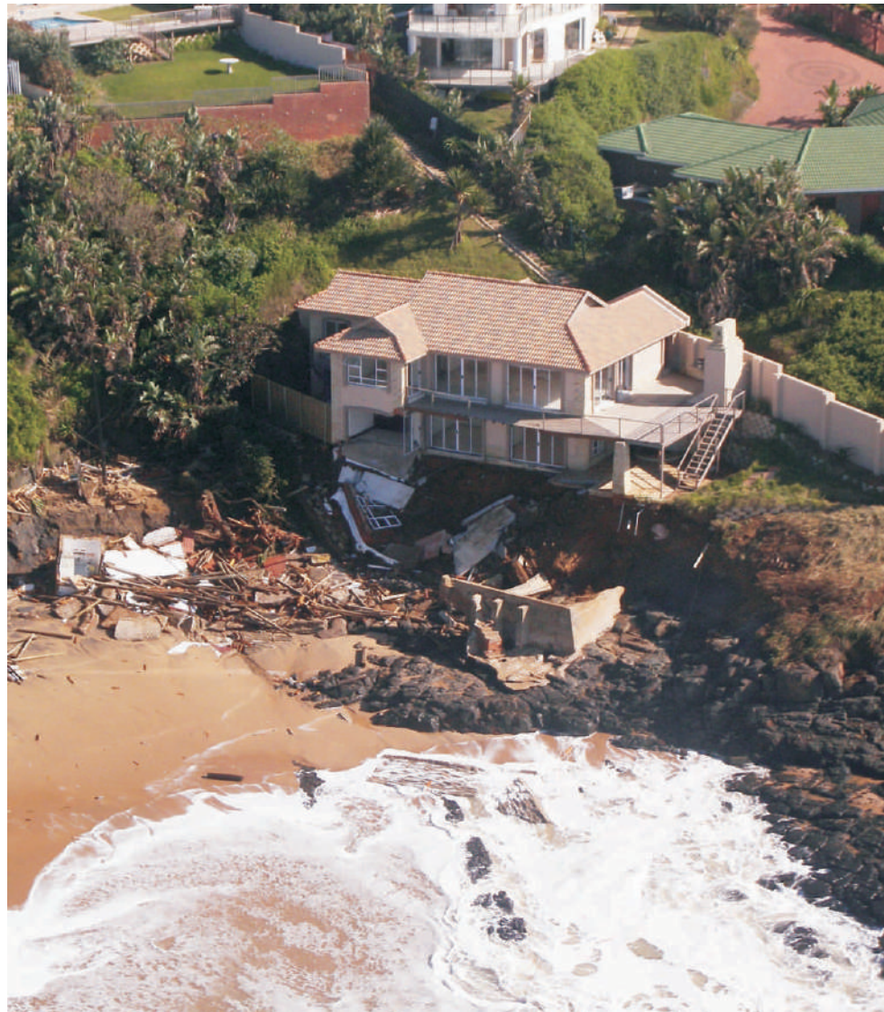
Damage to property as a result of an unusual climatic event.
