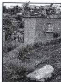
Vetiver grass used to protect a low-cost house in an urban setting
